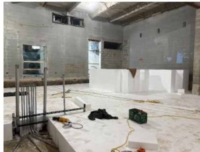
Geofoam under New Auditorium Floor Slab
