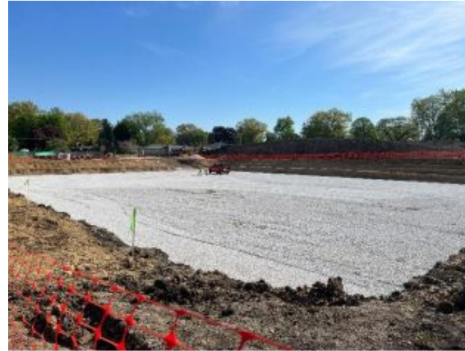
StormTrap Excavation & Stone Base
